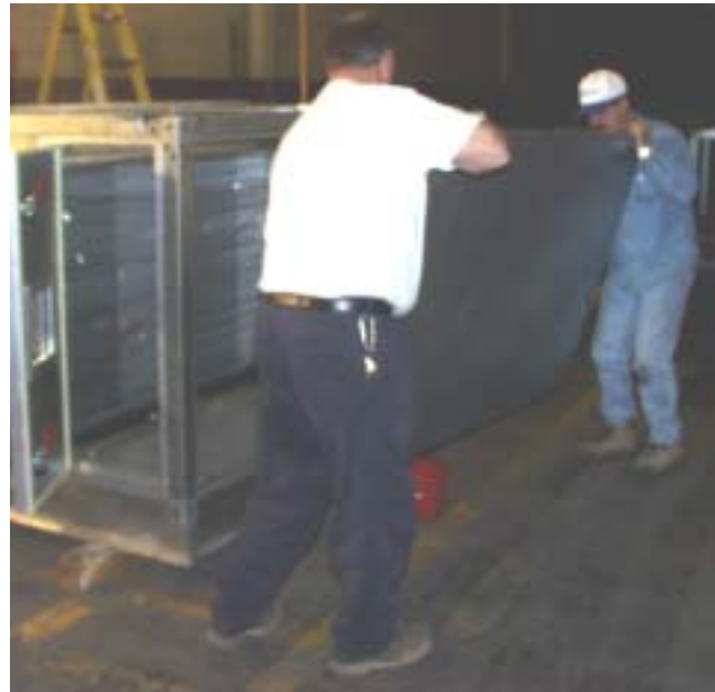
FIG. 14 - REMOVE LOWER BACK END PANEL(S)
