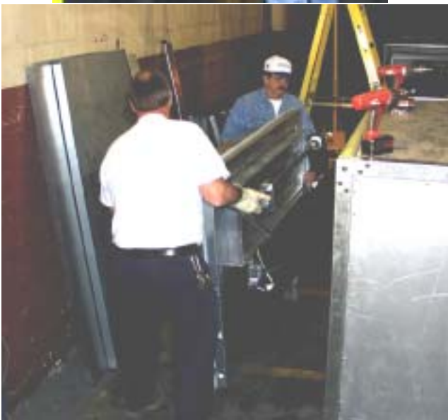
FIG. 13 - REMOVE BOTTOM FRONT END PANEL(S)
