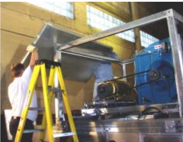
FIG. 6 - REMOVE TOP PANELS
