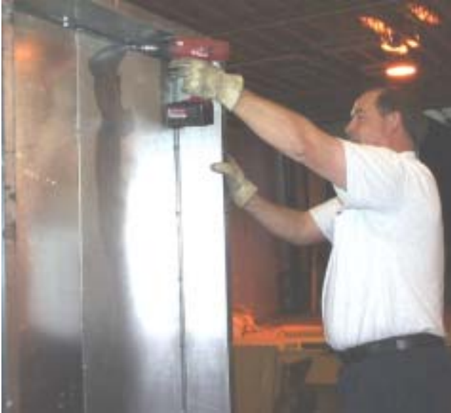
FIG. 27 - REMOVE SCREWS FROM BOTTOM OF FLOOR PANEL(S)
