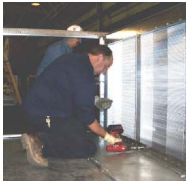
FIG. 18 - REMOVE SCREWS SECURING COIL
