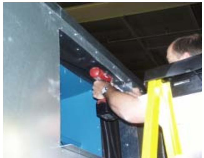
FIG. 4 - DISCONNECT FAN DISCHARGE FLEX CONNECTOR
